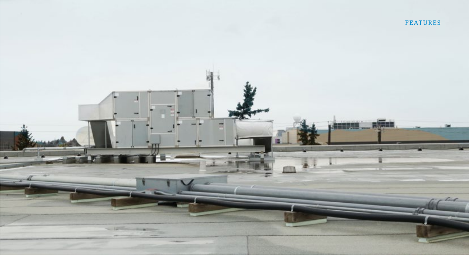
Heat reclaim units installed on the North Academic Building. Heat is recovered from the building's exhaust at a rate of up to 90%. On a one-degree day, the units bring in fresh air at 17 degrees!
